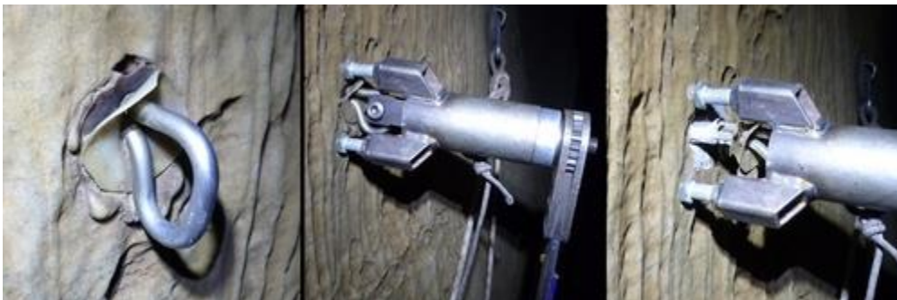
Removal of a loose DMM anchor installed in the early 1990s.
