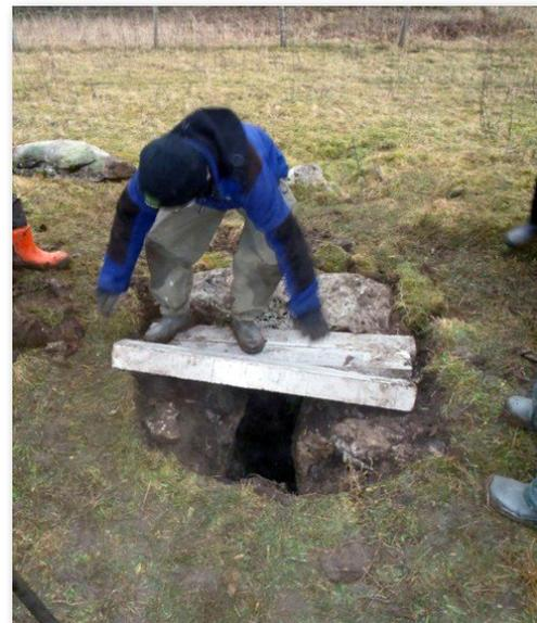
We also found the original Blood Cave entrance close by, directly under the track, covered by slabs and turf. The slabs and turf were replaced, and the other hole was made stock and tractor proof with concrete beams and covered with turf. This work was carried out with the support of Natural England and Stories in Stone.
