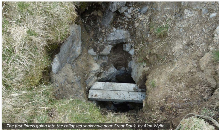
The first lintels going into the collapsed shakehole near Great Douk, by Alan Wylie
