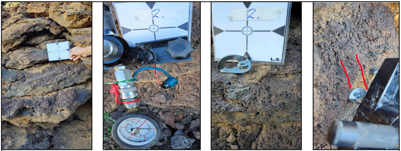
Fig. 5a, b, c and d, Showing location of test site 2, type of slab crusted lava flow, cracks and failure at 4kn
