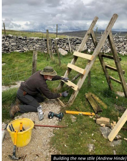
Building the new stile (Andrew Hinde)
