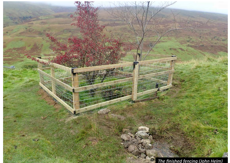
The finished fencing (John Helm)
