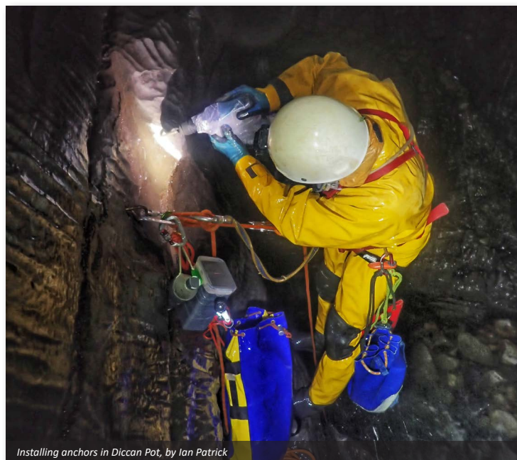
Installing anchors in Diccan Pot, by Ian Patrick
