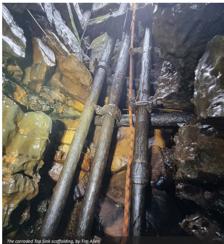
The corroded Top Sink scaffolding, by Tim Allen
