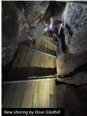
New shoring by Dave Gledhill
